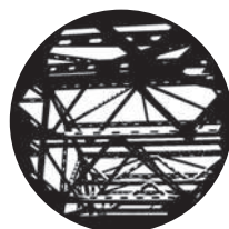
SR-6054 On A Bridge
